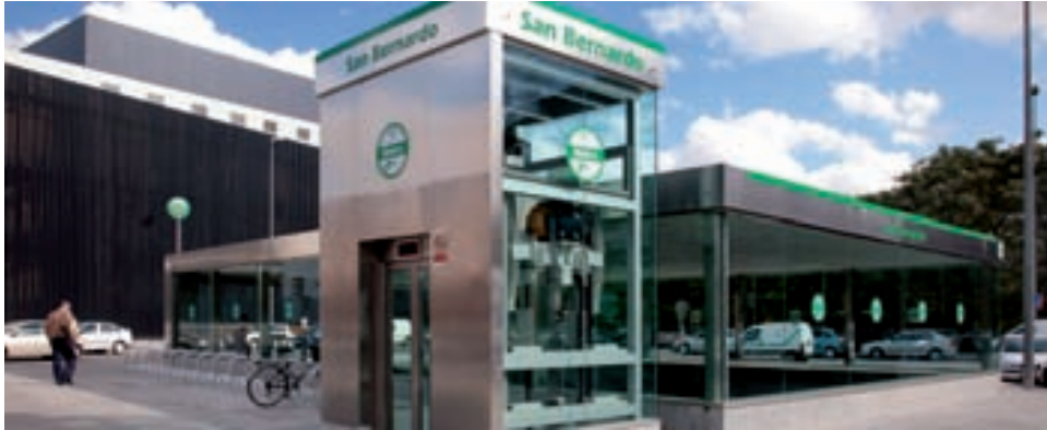
MP GLASS lift Seville metro. Seville. Spain.
